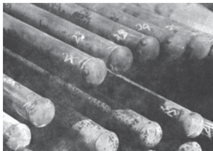
Case 69 (a) Schematic of the bottom portion of waste heat boiler. (b) Schematic of the concentric steam generator tube assembly with the bottom closure cap. (c) Photograph of damaged gas distributor. (d) Affected steam generator tube bundle with closure end caps at the bottom ends. (e) Steam generator tubes with blisters on the closure end caps.
