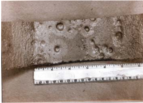
Case 38 Pitting corrosion due to dissolved oxygen in carbon steel boiler tube.
